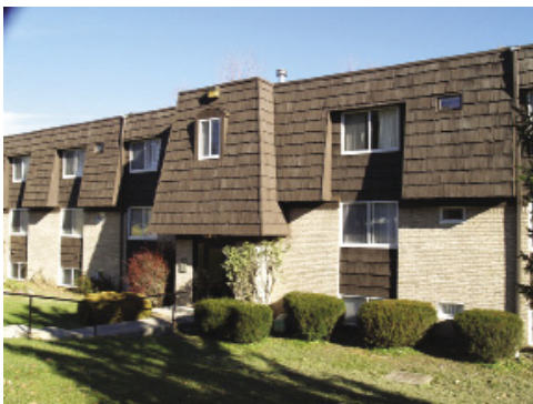
Fairmount Hills, 32 Lakeview Drive - Lakewood, NY
