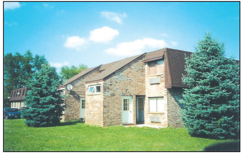
Northtown Apartments, Holland
