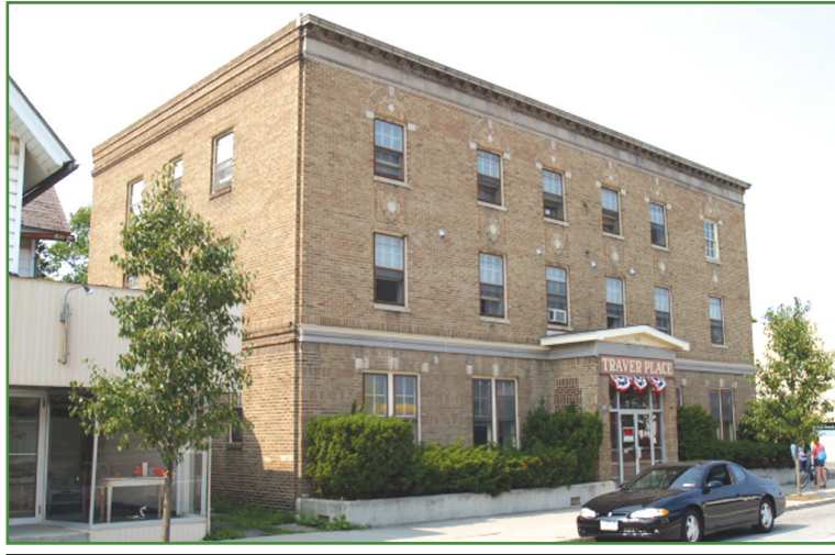
Traver Place Apartments, 55 South Main, Perry
